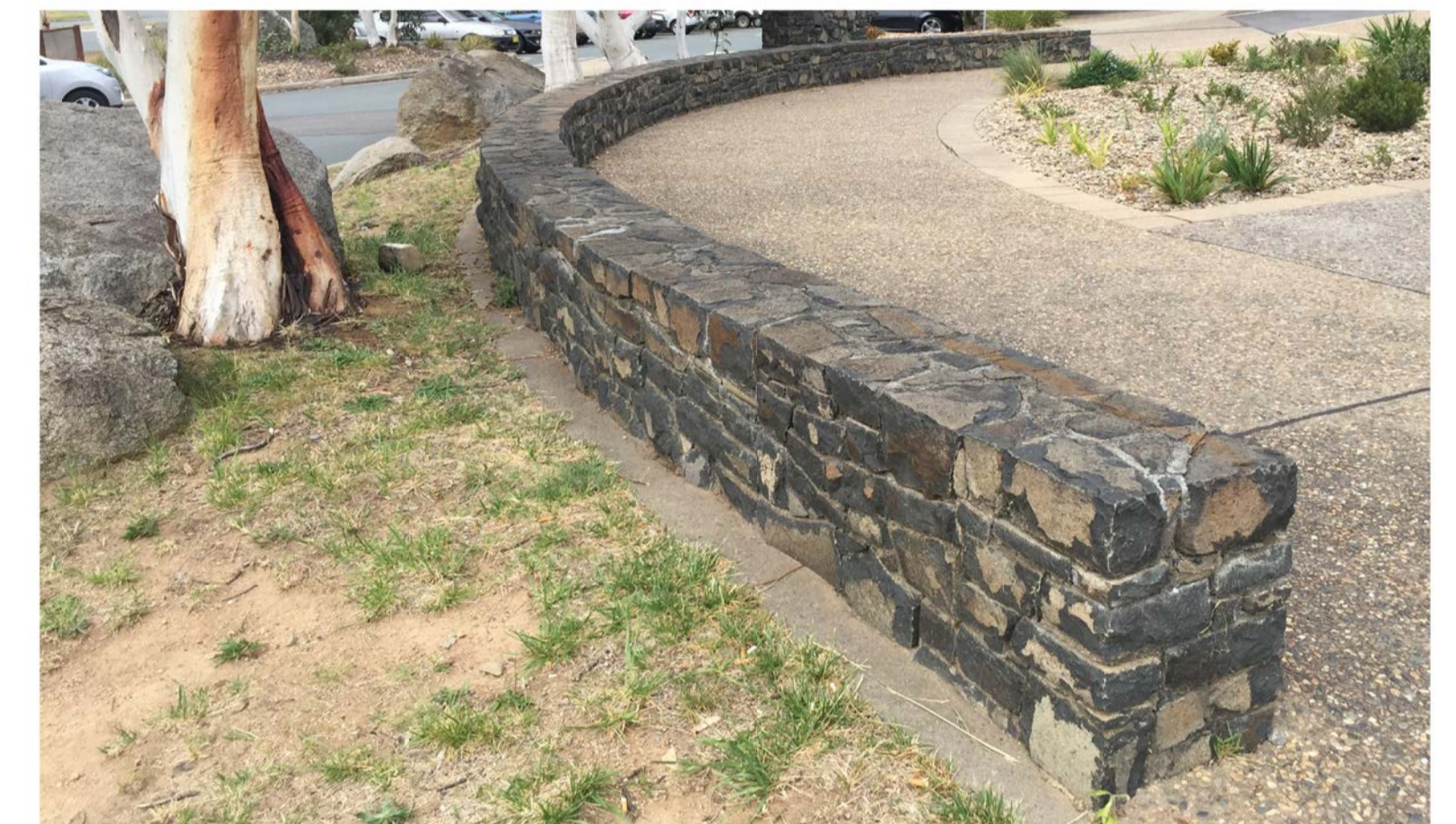
LOW STONE WALLS FEATURING LOCALLY SOURCED STONE MATERIALS
