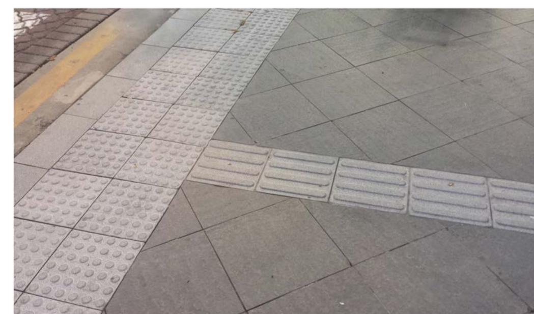
URBAN STONE TACTILE TYPE 'A' AND TYPE 'B'
