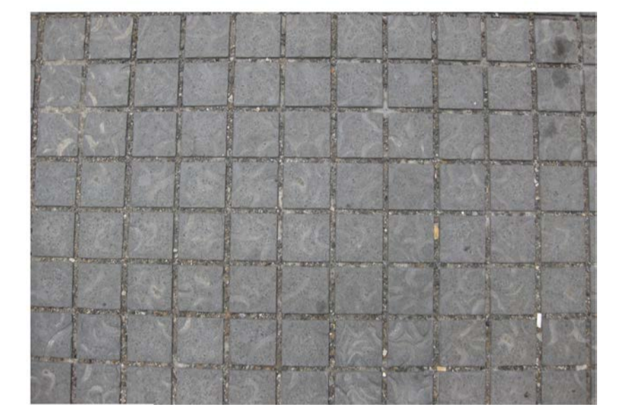
URBANSTONE 'COBBLE 6 IN 1' PAVING WITH CONTRASTING TEXTURE TO SIGNIFY ENTERING A DIFFERENT ROAD ENVIRONMENT AND CALM TRAFFIC
