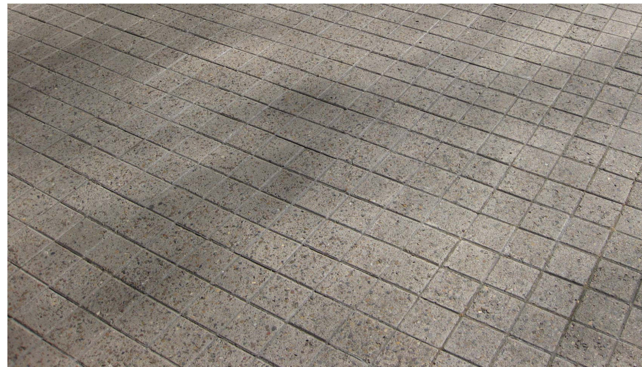
SHOTBLAST ADBRI BIPAVE FOOTPATH/ DRIVEWAY
