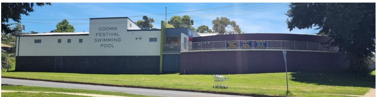
Figure 2: The southern view from the town or Massie Street.
