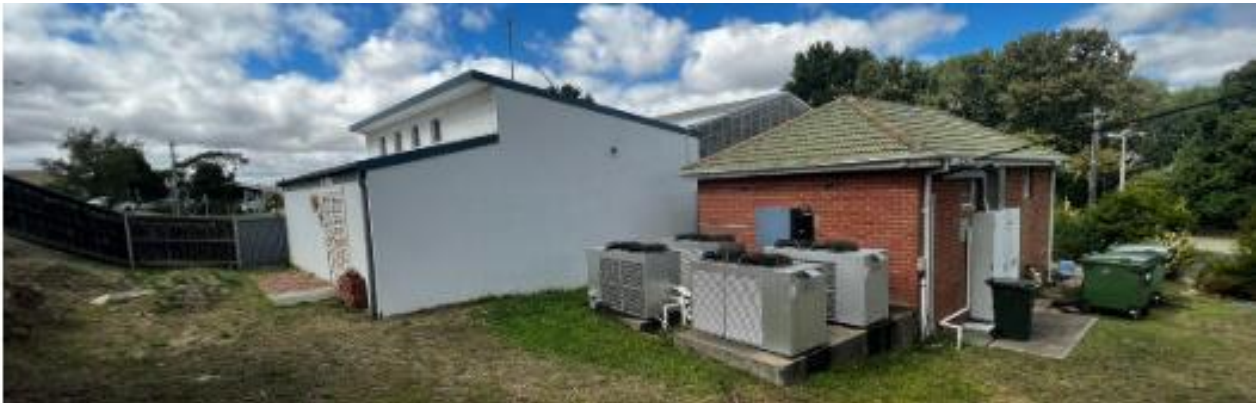
Figure 13: The current pump room as viewed from Crisp Street.
